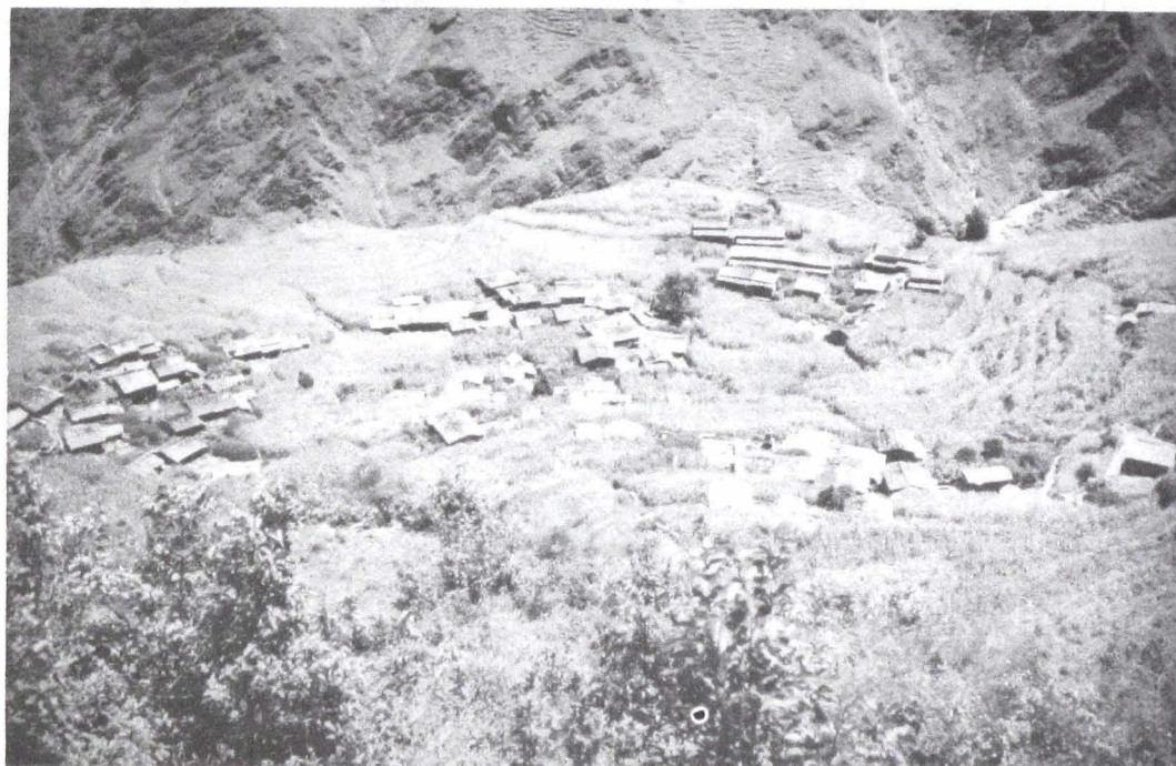
Figure 2.3. A View of Timling from the Southwest Ridge. Clearly visible are the clan neighborhoods: Damrong Tol in the lower right; Ganglememe in the upper right; Gangden to the extreme left; and Chetden near the tree in the center. This narrow shelf of land stretches from about 6500 ft. in elevation near Gangden to about 6800 ft. near Damrong Tol. The Timling Gompo, not visible here, is at about 7000 ft. on the hill to the right of Damrong Tol. In the valley below the village is the Dungsol Khola.
